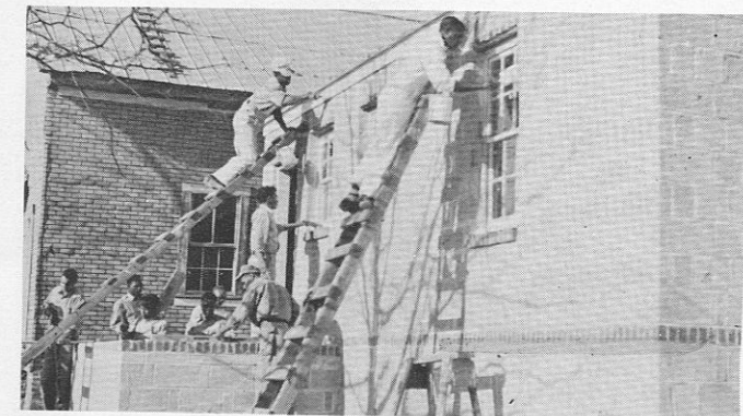
RURAL HOUSING COURSE - Trains Students in Agriculture in Low-Cash-Cost Construction with Concrete Blocks Made on the Farm
