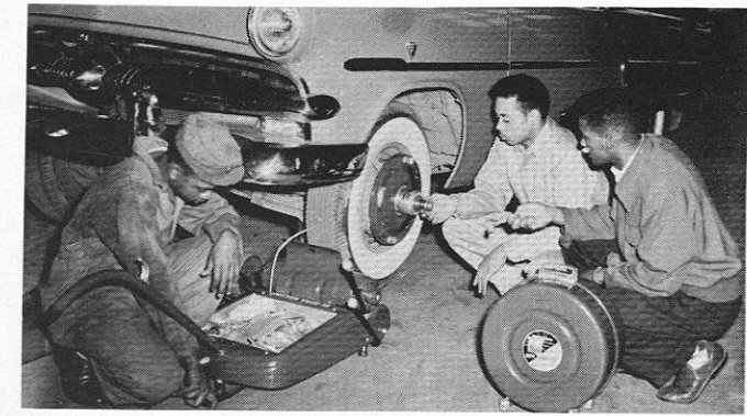
AUTO MECHANICS STUDENTS-Wheel Alignment Project
