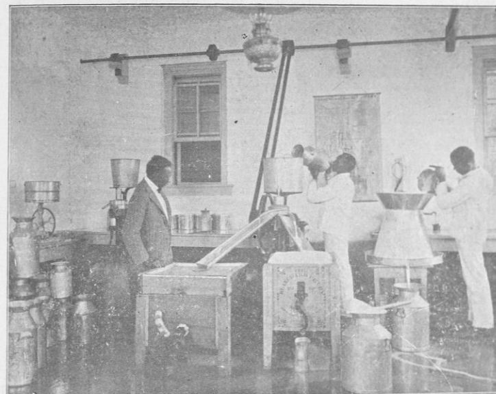
In the Dairy Room
