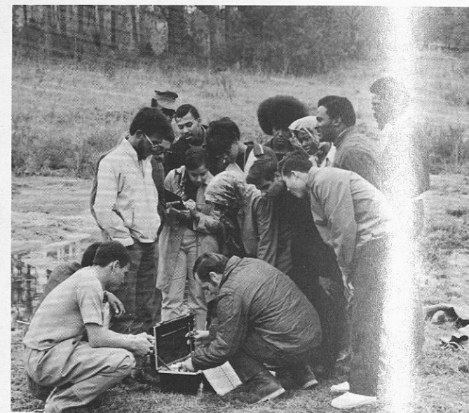
Improvisation is a necessary took of the modern biologist. Here, students make use of field equipment to accurately determine the oxygen content of a polluted water sample.
