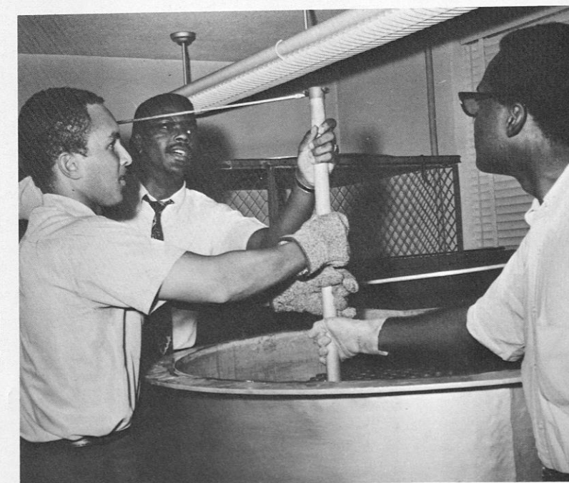
Engineering Students load natural Uranium fuel into a subcritical assembly.
