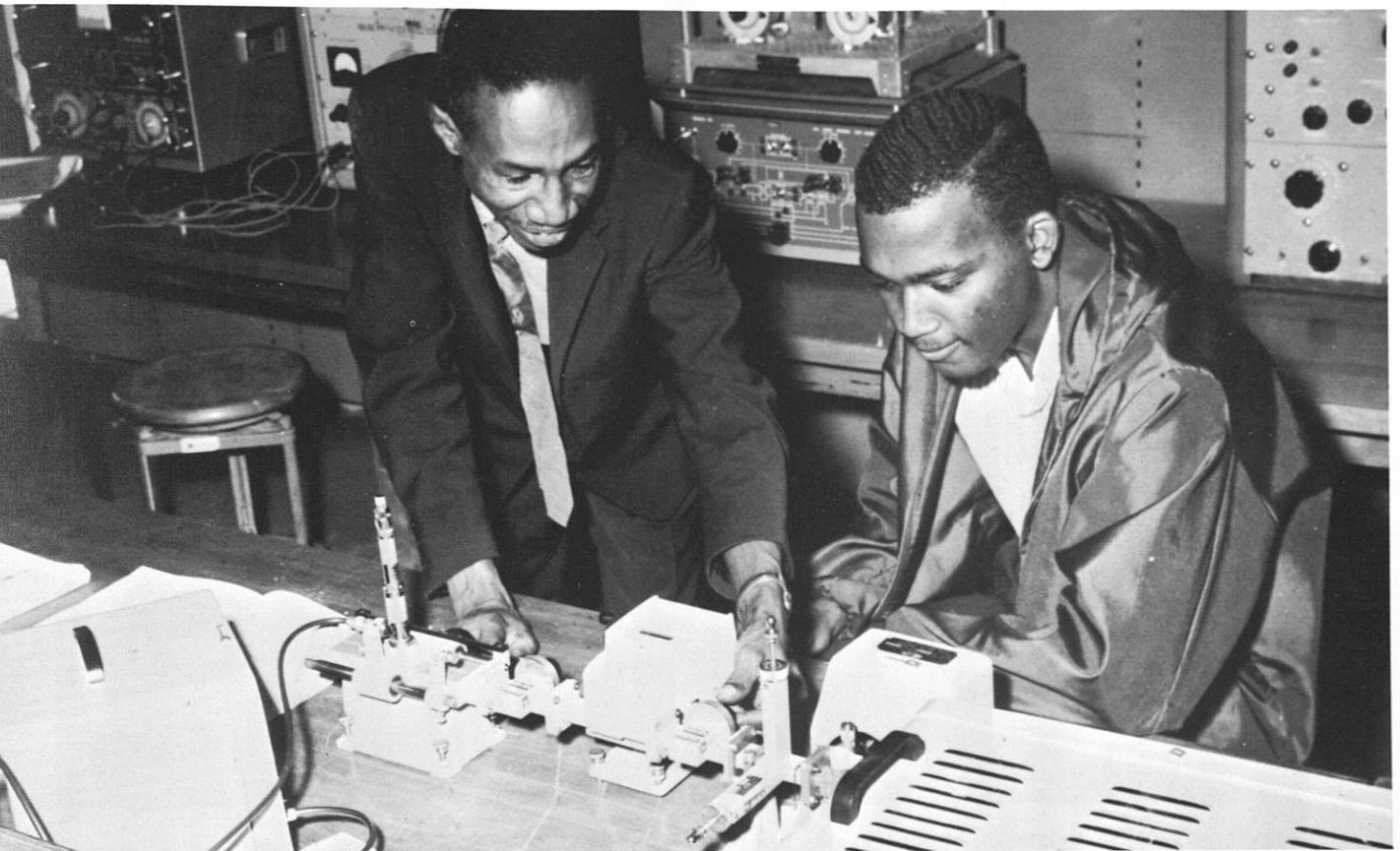
Mr. Britton—a staff technician sets up a waveguide apparatus for the electronics experiment.
