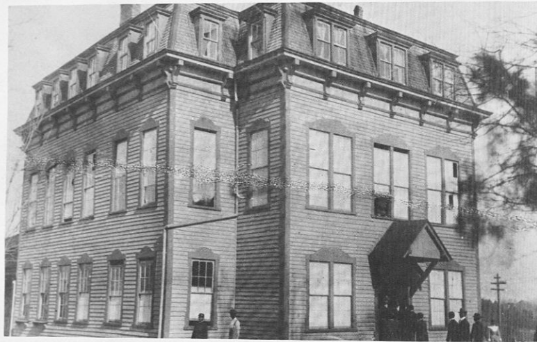
Porter Hall, schools' first building.
