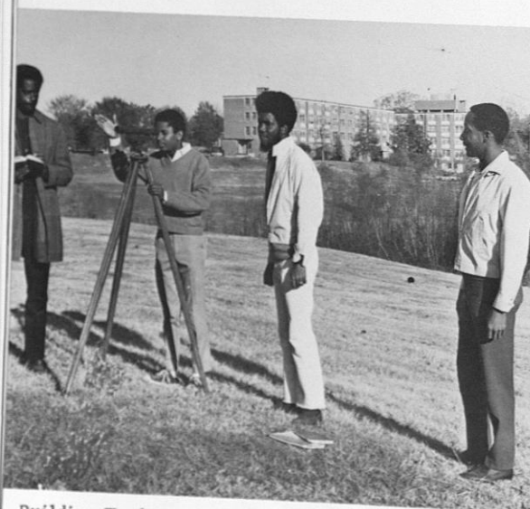
Building Technology students use surveying instruments to obtain land contour measurements.
