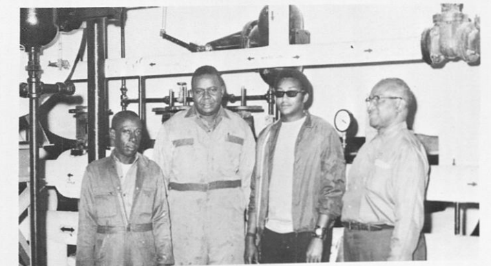
Power Plant, Left to Right: Lovie Crawford, John Milbry, Alonza Kennebrew, and Eugene Wynn, Supervisor Plant Operations.
