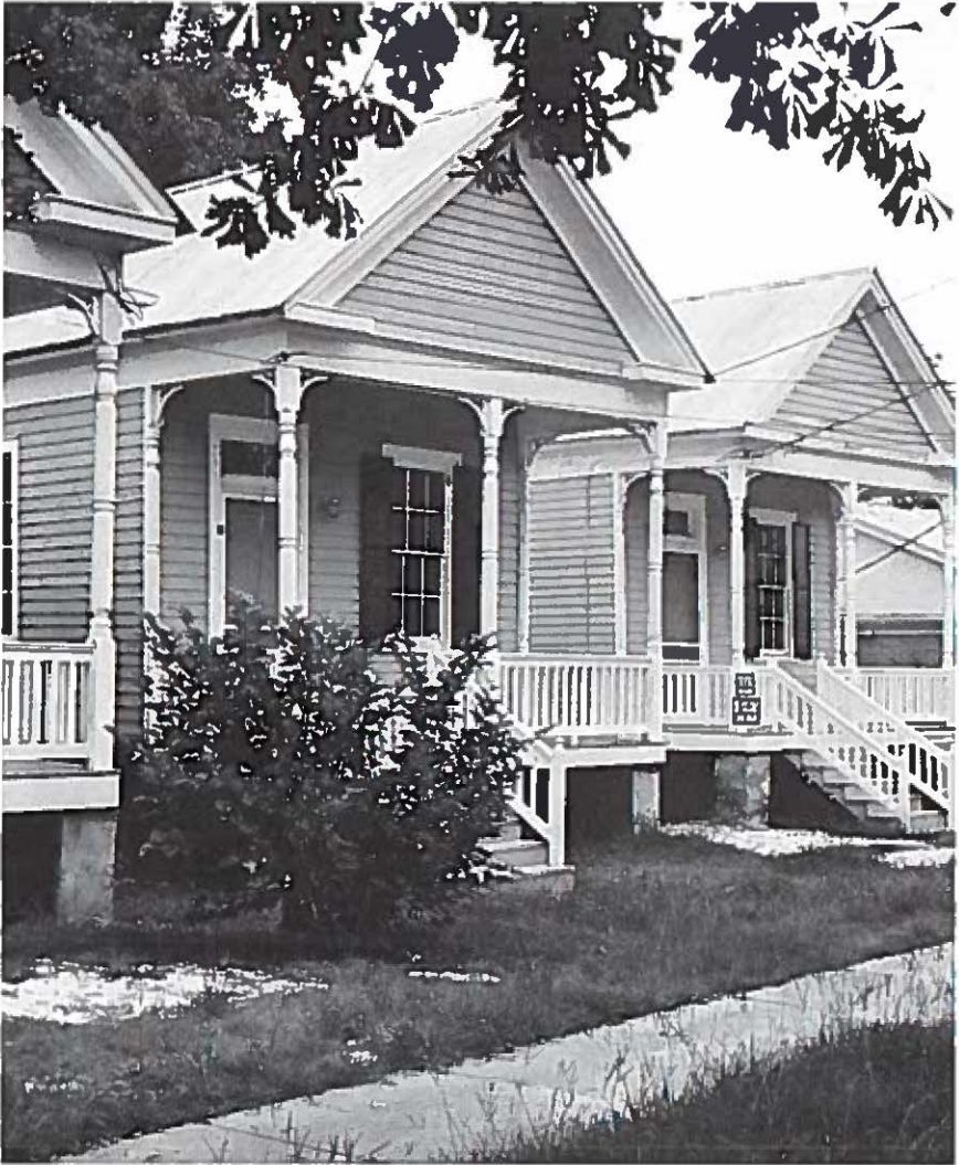
Renovated shotgun houses on Caroline St., 1990
