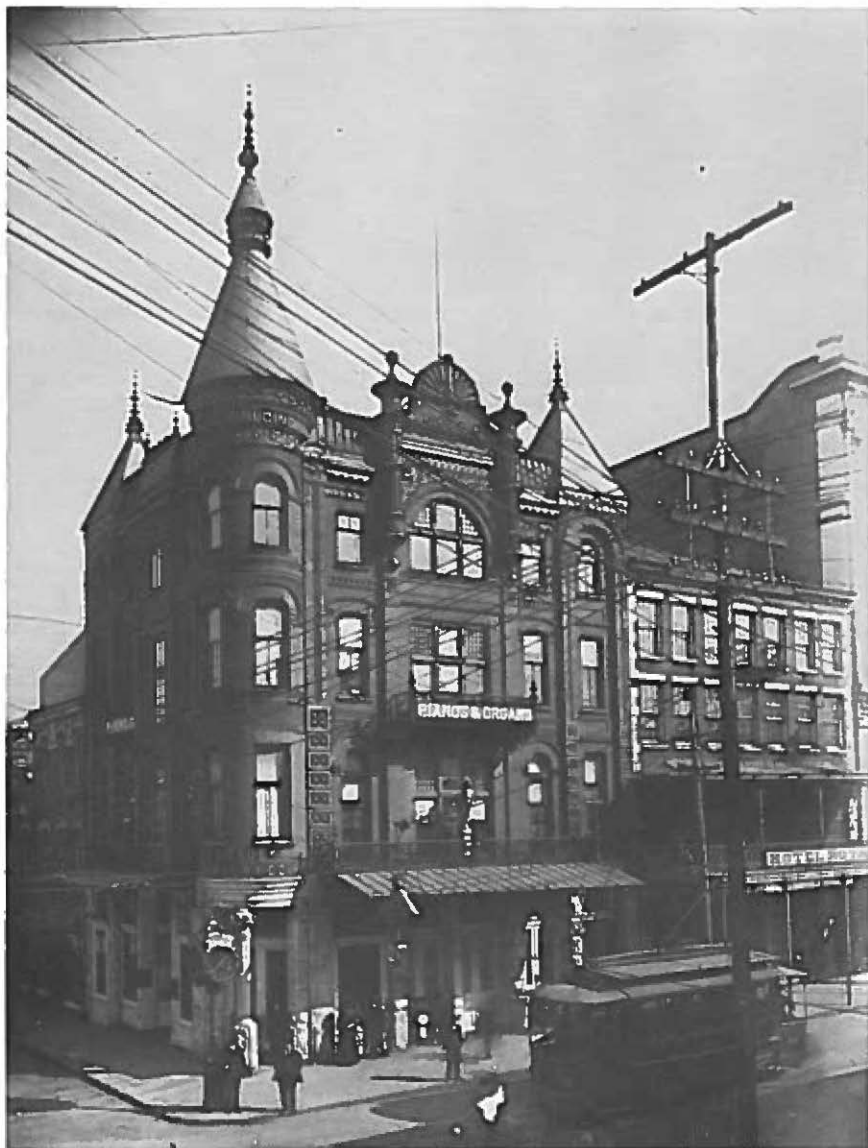
21. The Pincus Building (1890), southeast corner of Dauphin and Royal. The building was originally occupied by the Zadek Jewelry Company. A Victorian design in brick and terra cotta, with cast iron columns and balcony.
