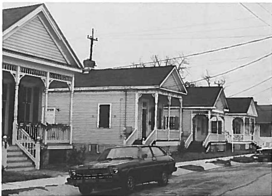
24. View of the west side of Cedar Street between Monroe and Eslava, showing cottages ranging in date from 1887 to 1905.
