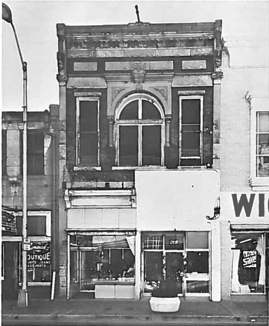
17. The Scheuerman Building (1893), 203 Dauphin Street. A. Kling, ironwork. This Victorian design in Philadelphia brick has trim of Alabama stone and granite columns framing the large central semicircular-headed window.
