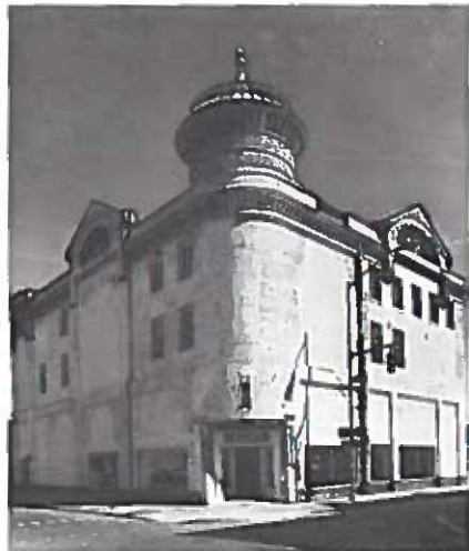
5. The German Relief Hall (1898). In the 1980 photo the windows and doors are infilled and plastered, only the main massing and the remarkable cornice remain in their original condition. The building on the corner of Conti and St. Emanuel Streets has been purchased for restoration. Its original appearance is suggested in the artist's rendering on the left based on an early engraving and photograph.
