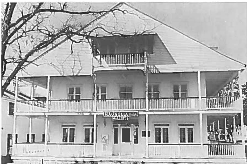
...and after restoration
