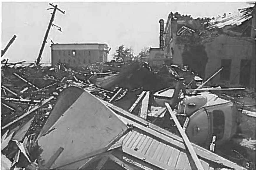
Water borne debris, Pass Christian
